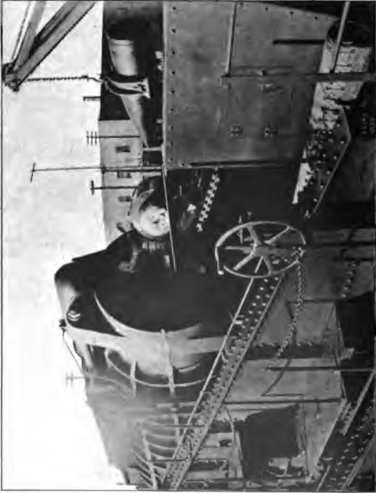
LOADING TABLE AND TRAY OF THE 12-INCH, 36-CALIBER AMERICAN GUN MOUNT.
